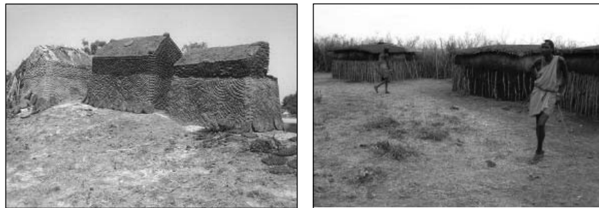
Architecture of minimalism: cow dung as fuel, India (left); and as a building material in a Maasai manyata in Maasailand, Kenya (right).
